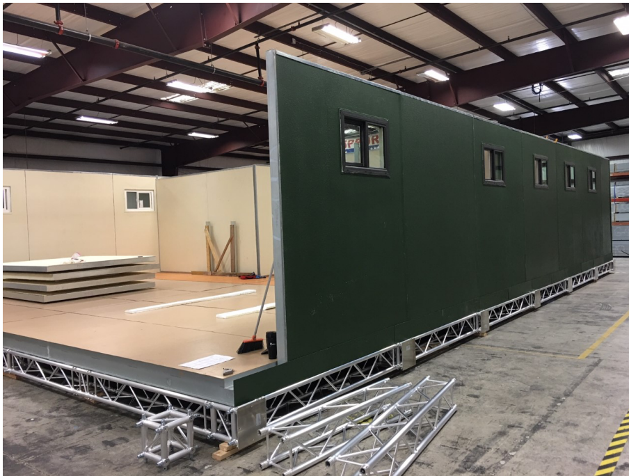
Photo 1: A readily deployable shelter being constructed at the WHS manufacturing site [9].
